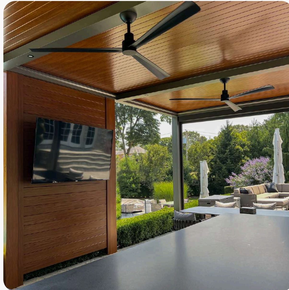
PRIVACY WALL without gap
